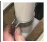
Pinch the bracket ends back together.
